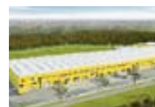
RO, Logistics centre Pantelimon
