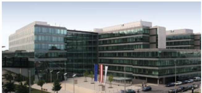
Office Campus Gasometer | Vienna | AT
