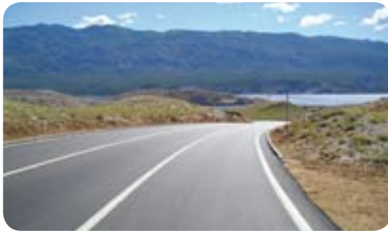
Approach Road to the Ferry Harbor Uvali Misnjak, Island of Rab, Croatia
