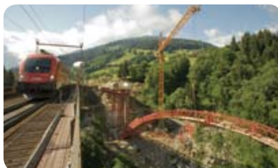
Railway bridge, Angerschluftbrücke, Bad Hofgastein, Austria
