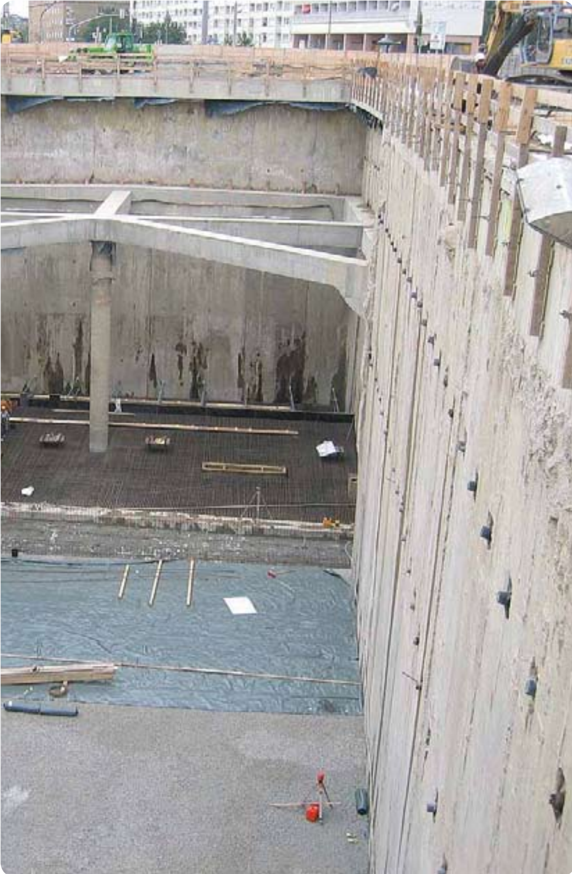
City tunnel, Leipzig, Germany
