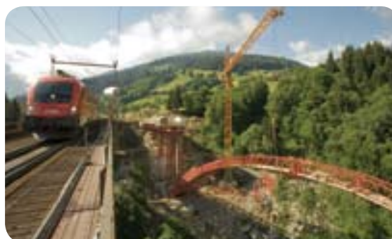
Railway bridge, Angerschluftbrücke, Bad Hofgastein, Austria
