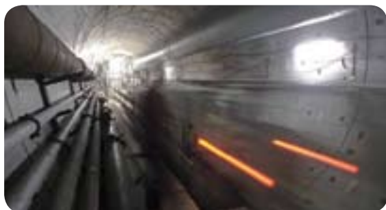
Staten Tunnel Randstad, Rotterdam, Netherlands
