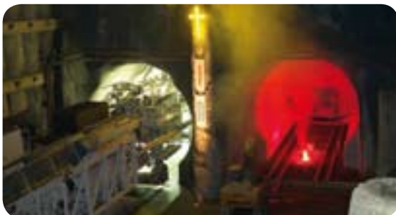
Railway tunnel, Gotthardbasistunnel, Erstfeld, Switzerland
