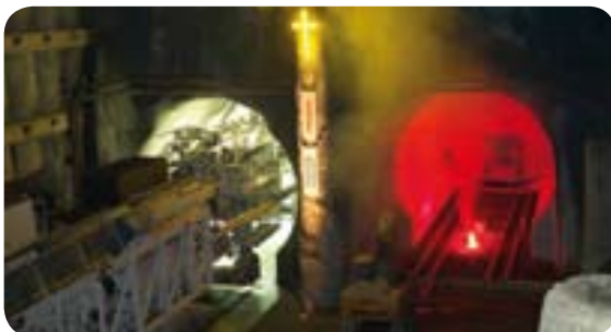
Railway tunnel, Gotthardbasistunnel, Erstfeld, Switzerland
