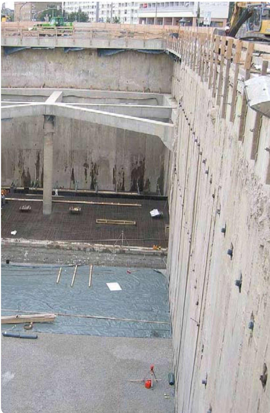
City tunnel, Leipzig, Germany
