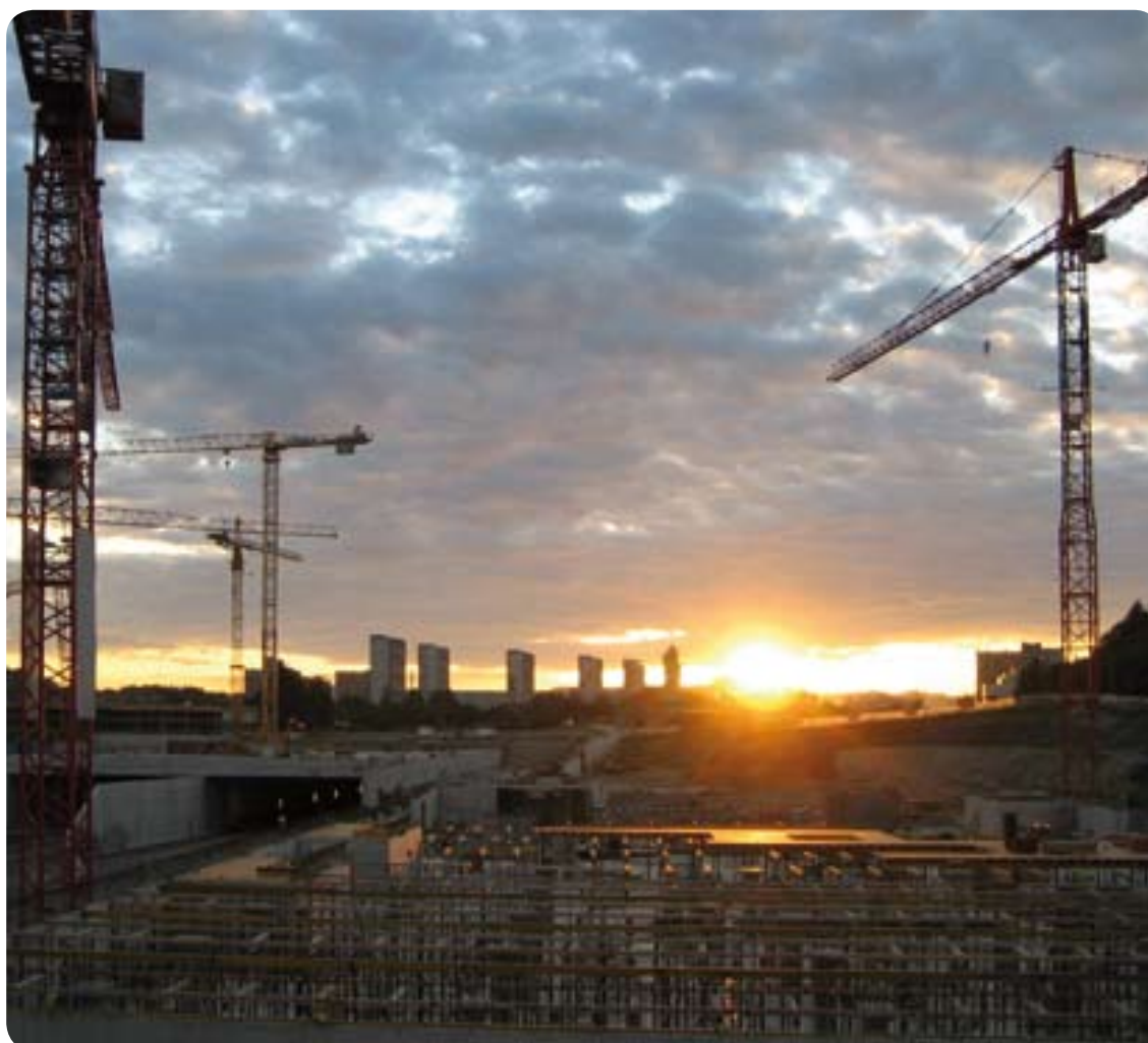
Leisure and shopping centre Westside, Bern, Switzerland
