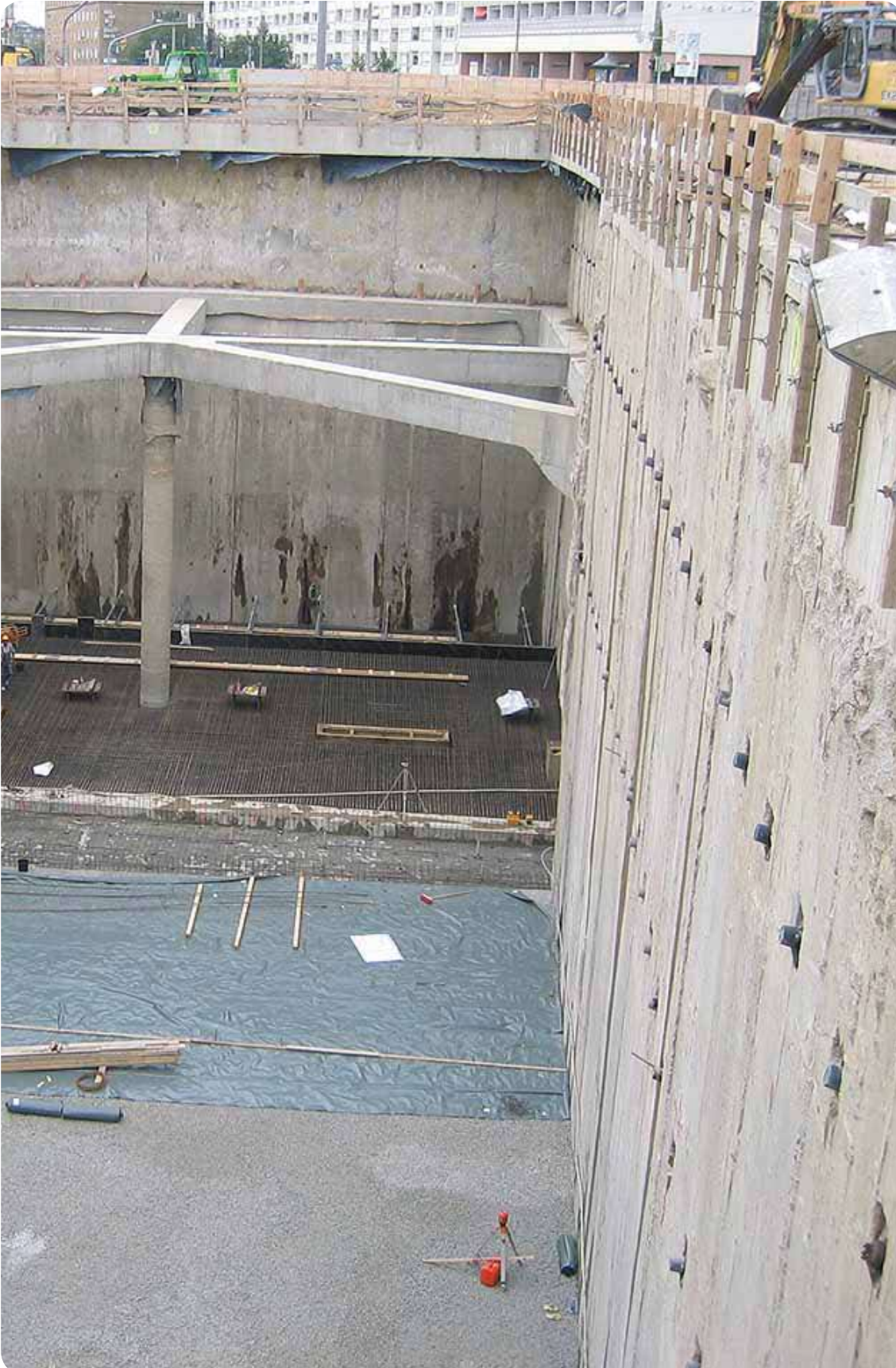
City tunnel, Leipzig, Germany
