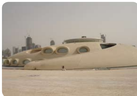
Private Beach Villa Project, Qatar
