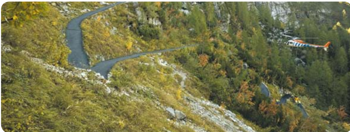
Bituminisation entry cavern system, Dachstein, Upper Austria, Austria
