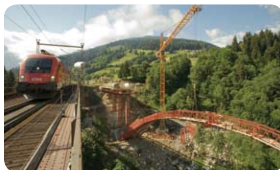
Railway bridge, Angerschluftbrücke, Bad Hofgastein, Austria
