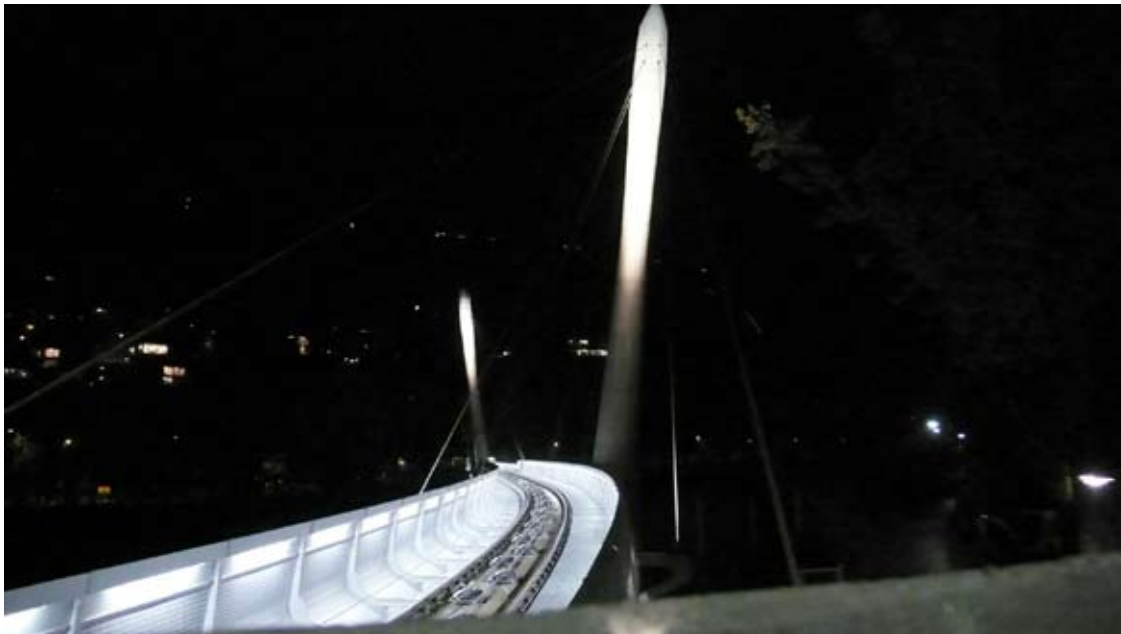
Project Hungerburgbahn, Innsbruck, AT Brand Zumtobel Realisation November 2007
