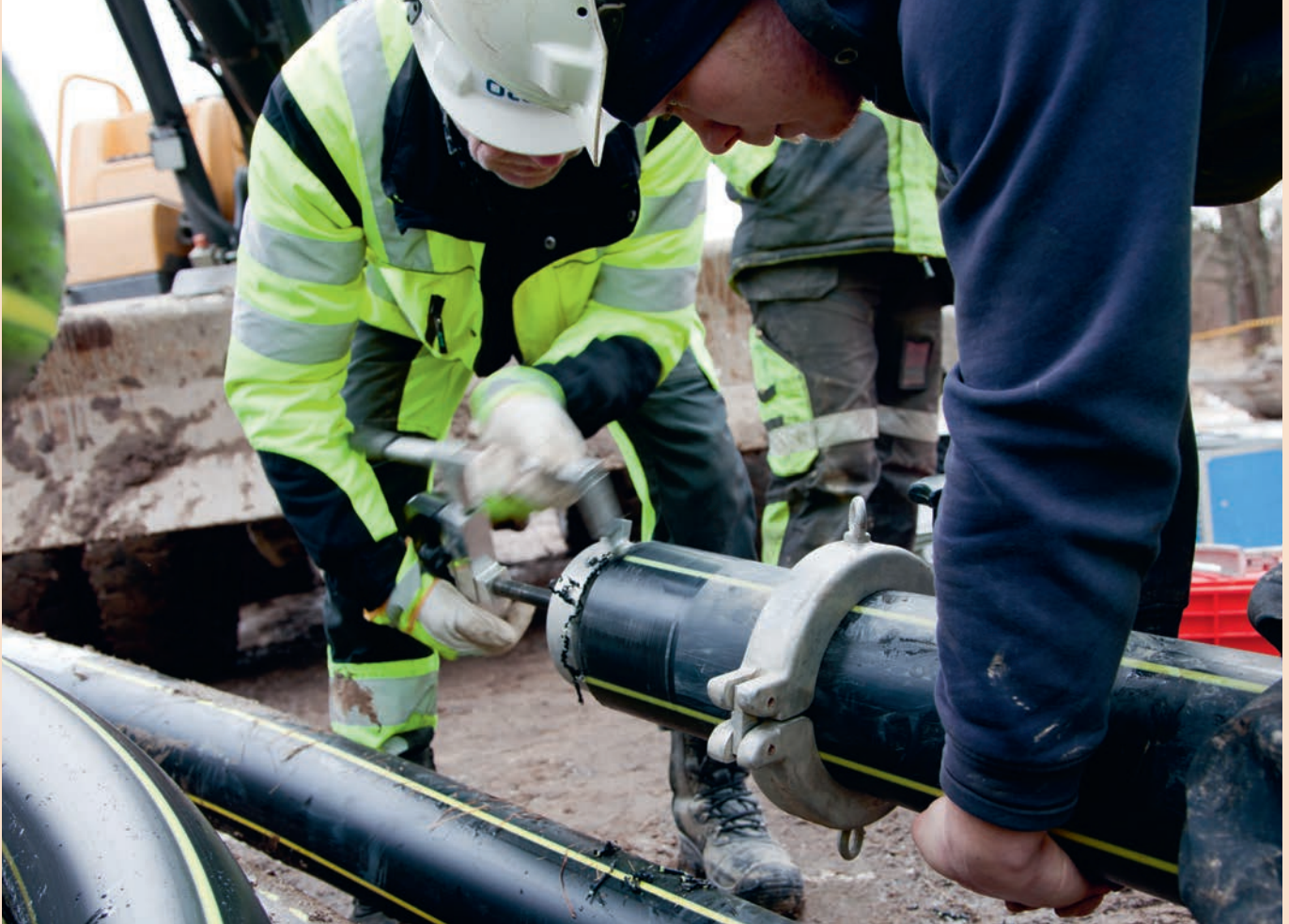
New laying technique for underground high-voltage lines
