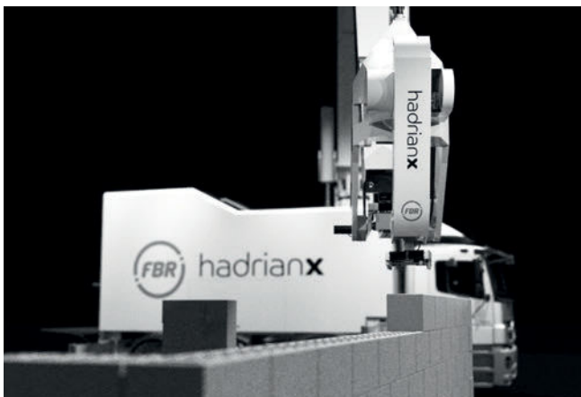
Robots at the construction site: Hadrian X erecting high-precision brick walls.
