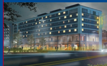
06/2009 Topping-out ceremony at angelo hotel in Katowice (197 rooms)
