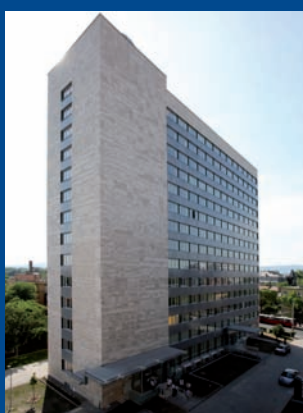
05/2009 Opening of Erszebet Office B, Budapest, after redevelopment
