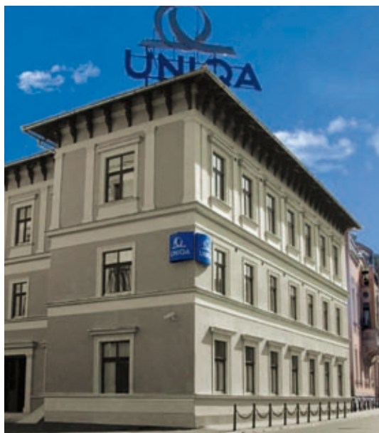
Since September 2009 the employees in Sarajevo have been working in a lovingly restored, historic student dormitory.
