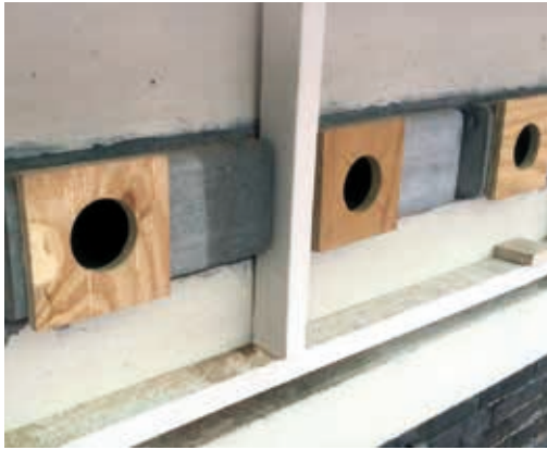
Nesting boxes integrated into the facade
