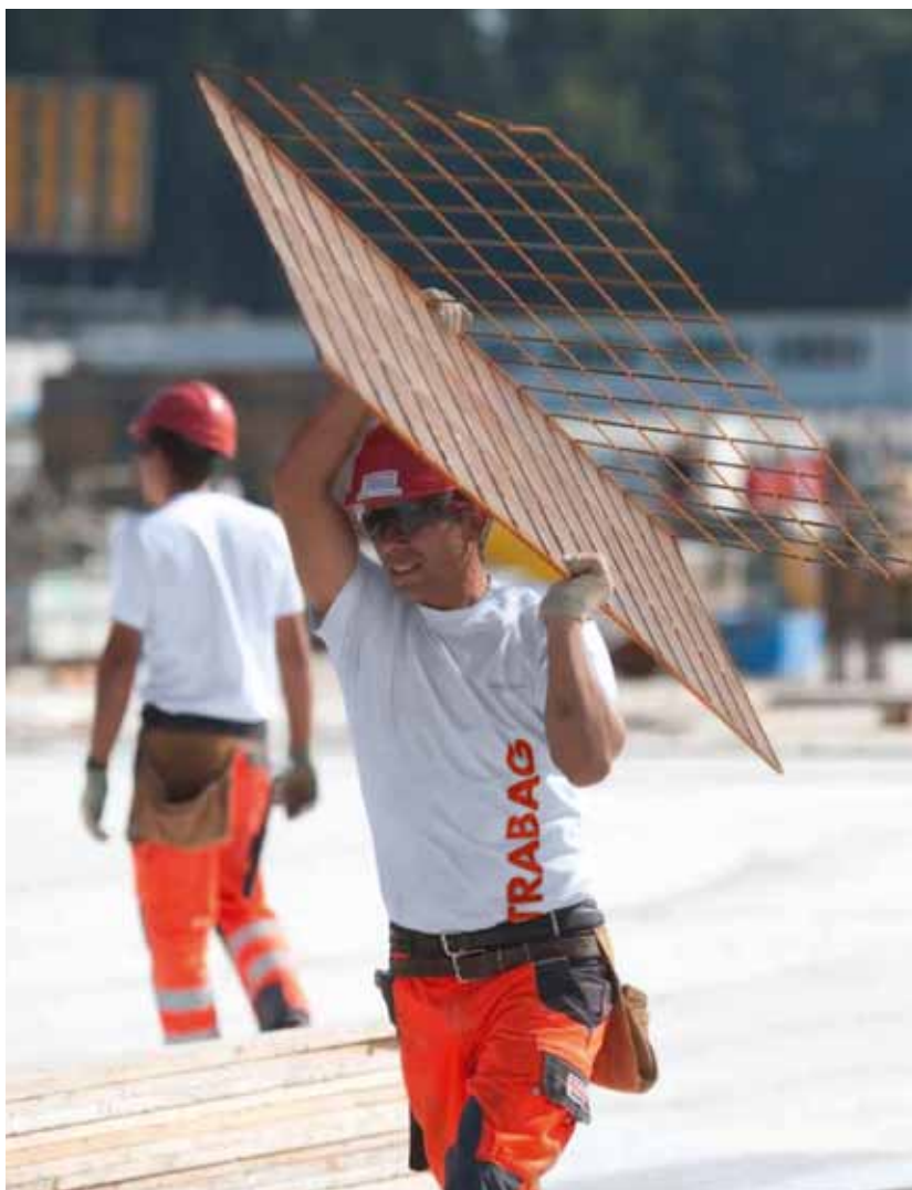
WORKS AT ALDI HEADQUARTERS, SWITZERLAND
