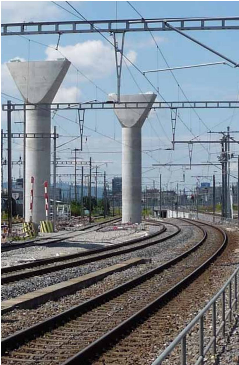
SBB BRIDGES, ZURICH CROSS-CITY LINK OERLIKON-ALTSTETTEN, ZURICH, SWITZERLAND
