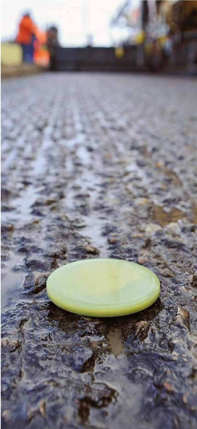
DATA TRANSPONDERS IN THE ASPHALT PROVIDE VALUABLE INFORMATION
