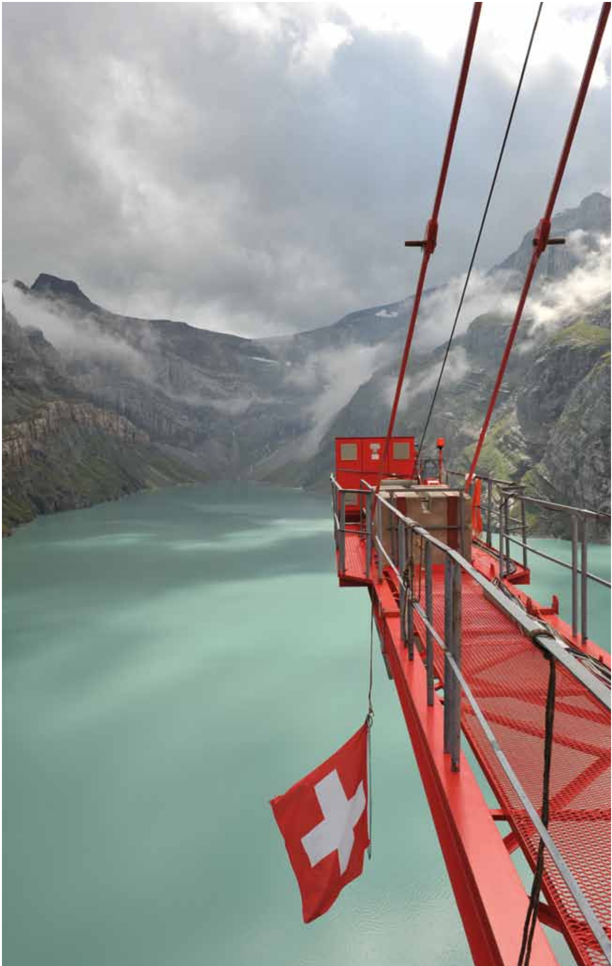
LINTH-LIMMERN MATERIAL ROPEWAY, SWITZERLAND
