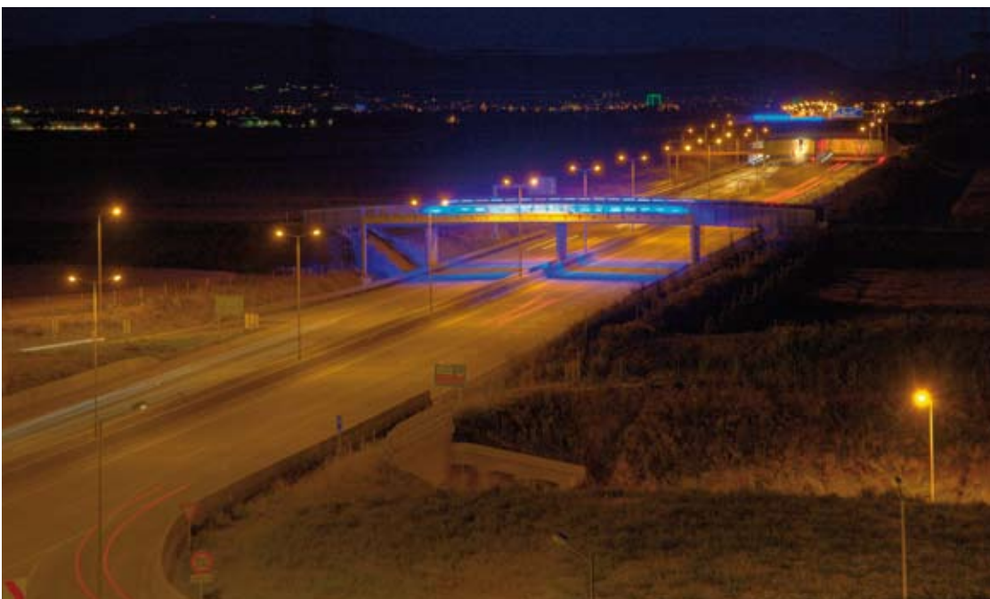
EXPRESSWAY S1, SCHWECHAT/RANNERSDORF, AUSTRIA
