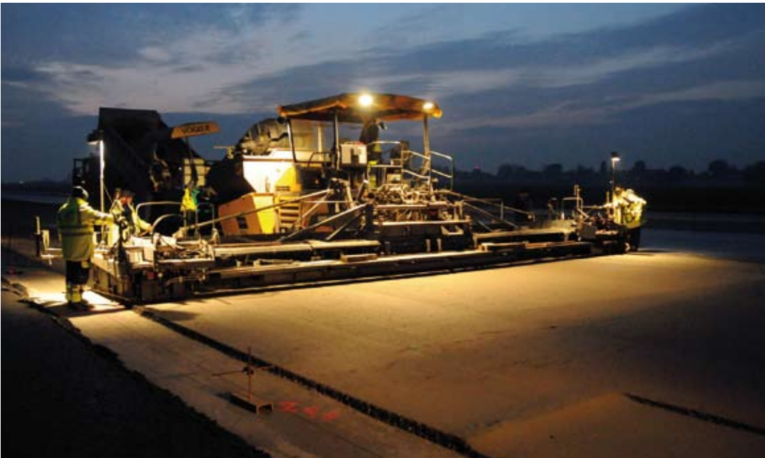
ASPHALTING AIRPORT KBALY, CZECH REPUBLIC
