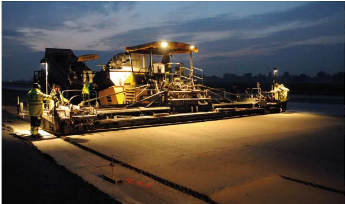
ASPHALTING AIRPORT KBALY, CZECH REPUBLIC
