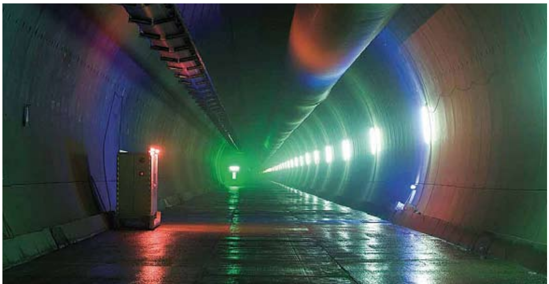
ISLISBERGTUNNEL, UETLIBERG WESTERN KNONAU, SWITZERLAND
