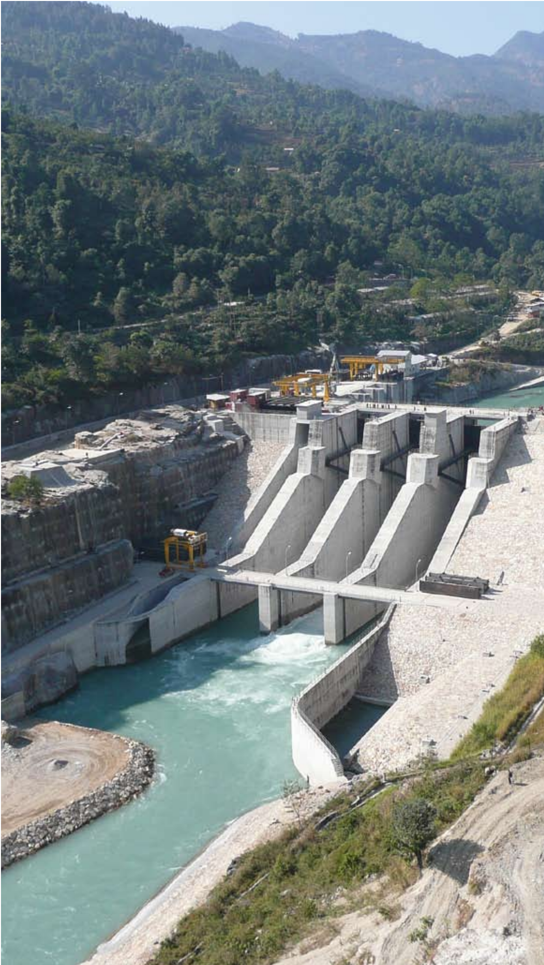
MIDDLE MARSYANGDI HYDROELECTRIC PROJECT, NEPAL
