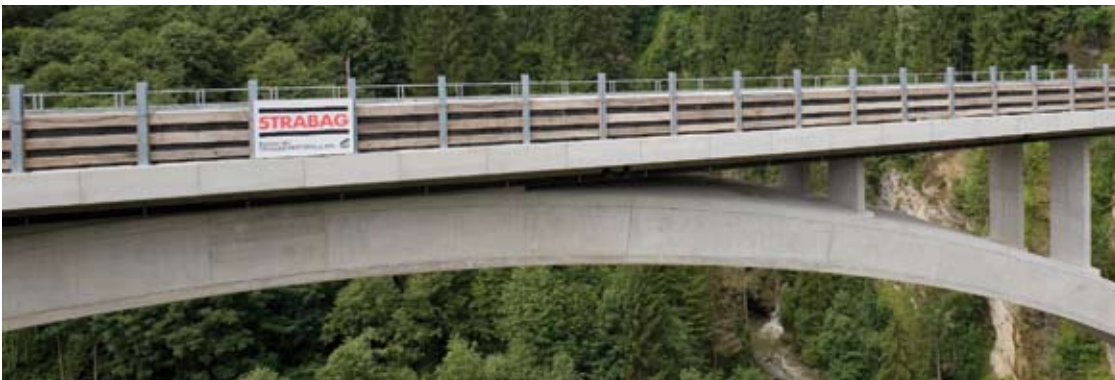
ANGER GORGE BRIDGE, BAD HOFGASTEIN, AUSTRIA
