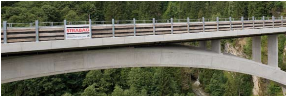
ANGER GORGE BRIDGE, BAD HOFGASTEIN, AUSTRIA
