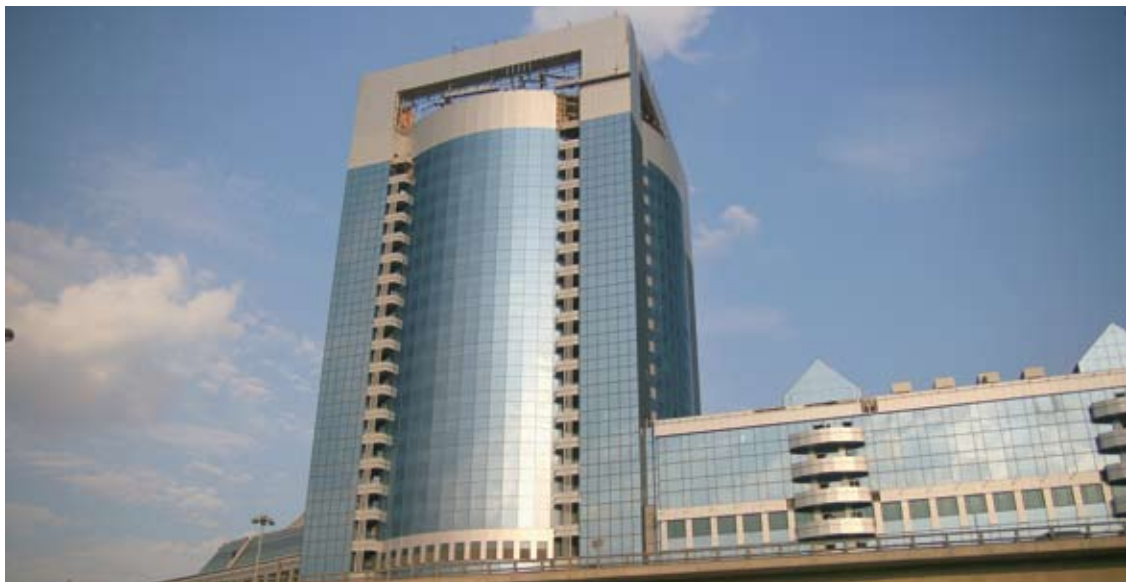
OFFICE BUILDING WITH PARKING “NORTH TOWER”, MOSCOW, RUSSIA
