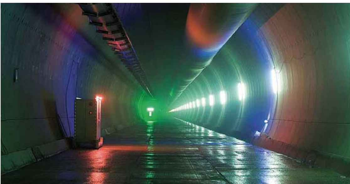
ISLISBERGTUNNEL, UETLIBERG WESTERN KNONAU, SWITZERLAND
