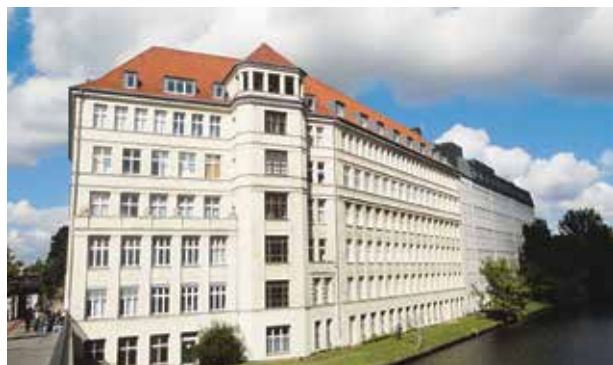
Office property Sonnenallee
