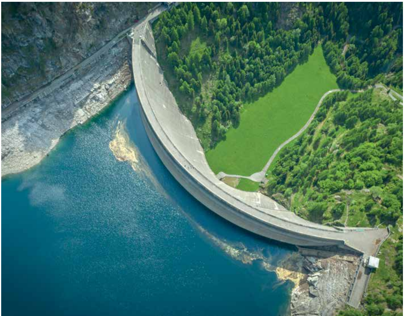
At the Mooserboden storage power plant in Kaprun, an intake and outlet structure separates the two existing dams at around 2,000 metres above sea level. The main challenge of this project was the large number of workstations, some of which were located in the high alpine region.
