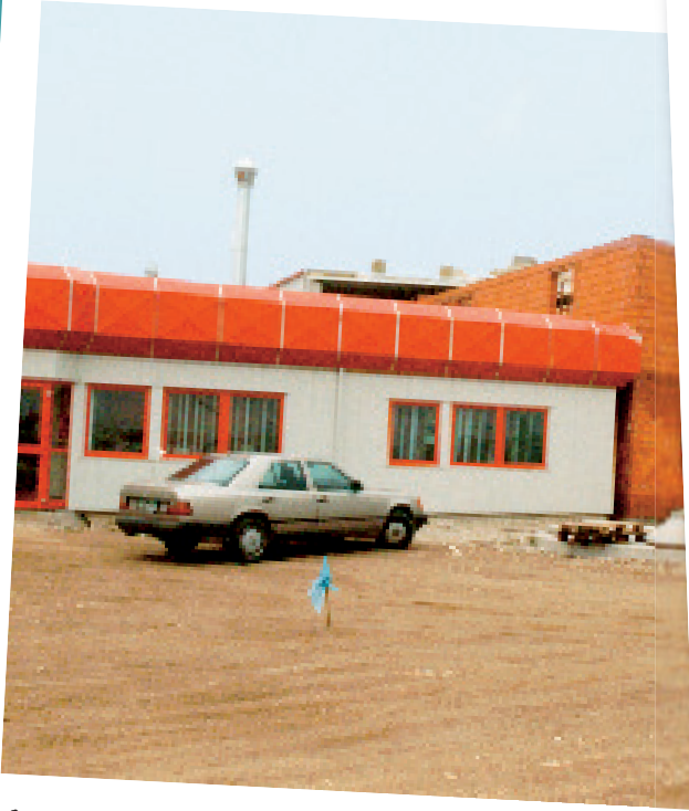
POLYTEC ELASTOFORM BUILDING UNDER CONSTRUCTION 1988
