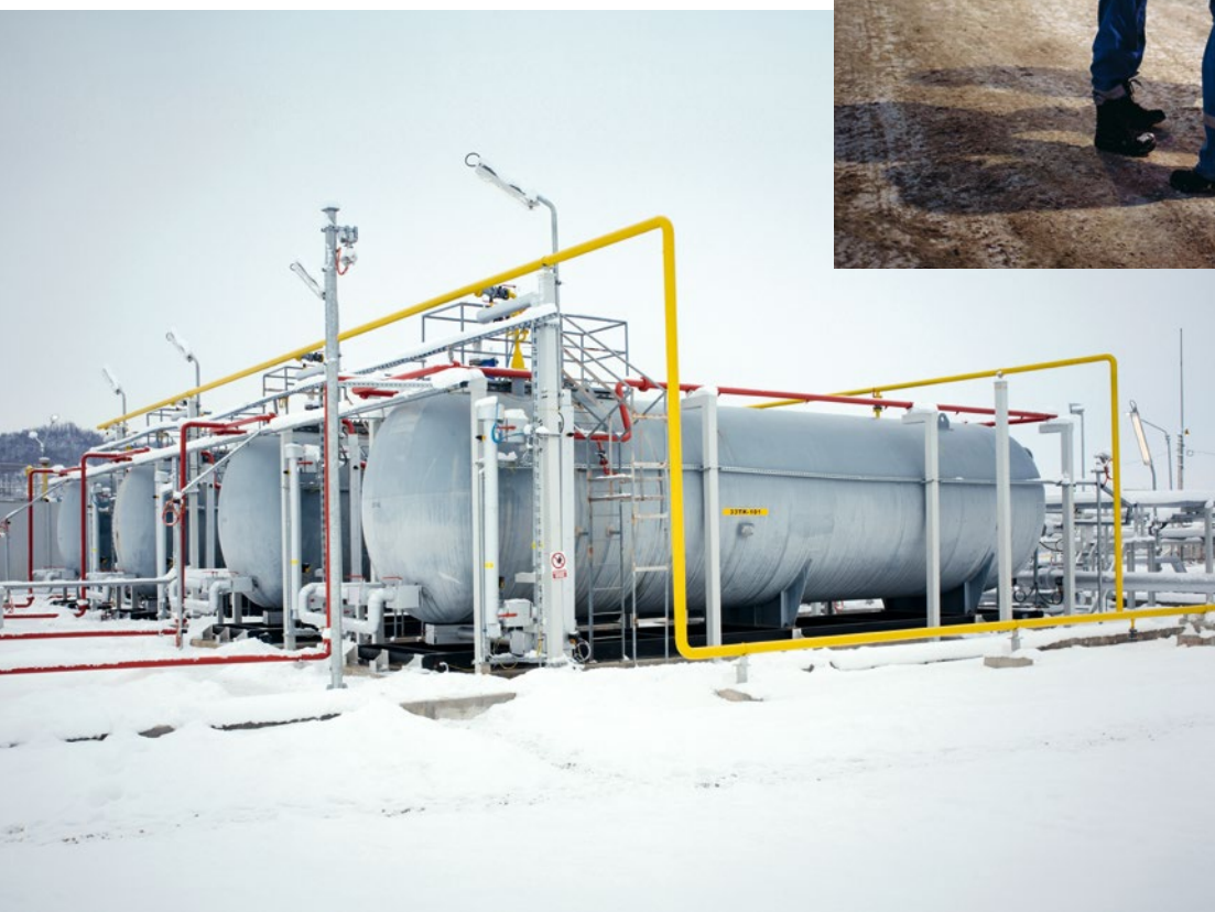
At the end of the day, all information is handed over to the night shift (top). Condensate storage vessels are positioned in a dyke for ultimate safety (left).
