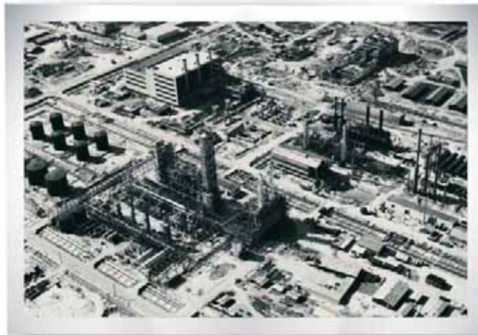
Schwechat refinery, on the outskirts of Vienna, shortly before recommissioning in 1960.
