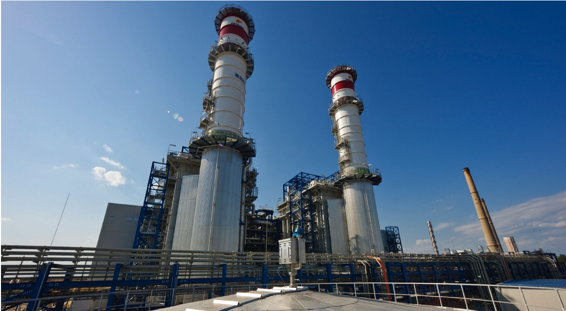
Power plant Brazi
