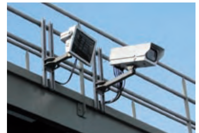
Automatic number plate recognition – ANPR
