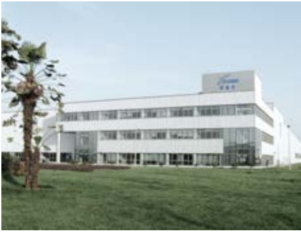
FACC developed the entire plant layout and specified the necessary equipment for its Chinese sister company Fesher.
