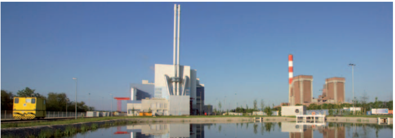
The power station and the waste incineration plant in Dürnrrohr form the starting-point of a comprehensive energy and infrastructure project.
