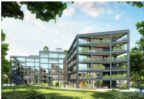
Grasblau is being developed by CA Immo as another fully digitized office building for efficient, healthy, safe and sustainable building operations
