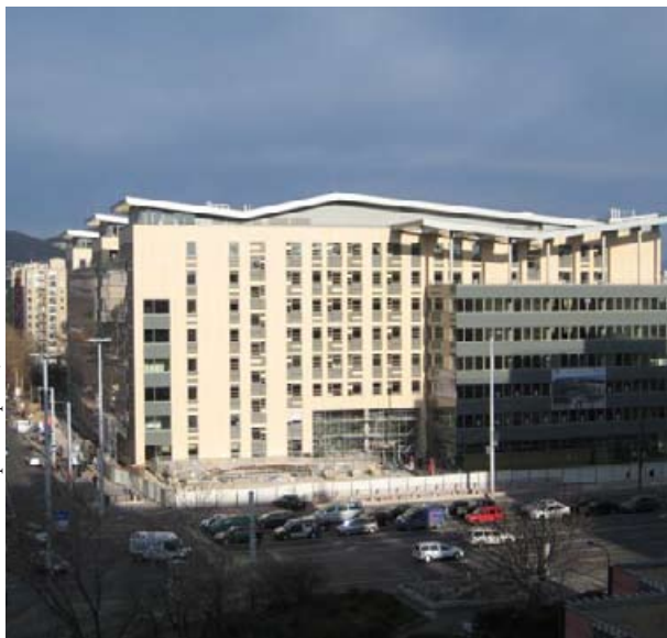
BUDAPEST Capital Square, construction site
