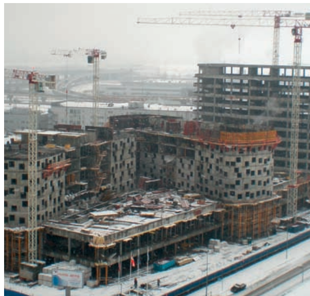
ST. PETERSBURG Airport City St. Petersburg, construction site
