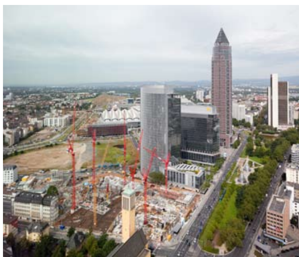
FRANKFURT Tower185 (Construction site) Entrance to the Frankfurt Europaviertel
