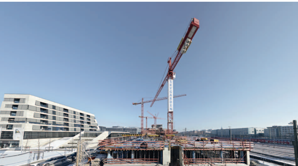
ARNULFPARK® Munich, construction site Skygarden
