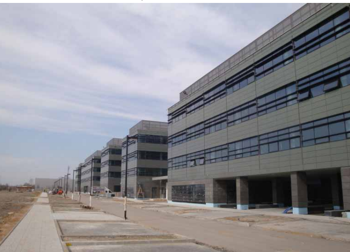
POLECZKI BUSINESS PARK Warsaw, Phase I finished
