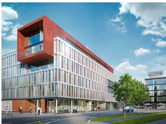
Office building Belmundo and Lavista in Düsseldorf: Start of construction in 2012
