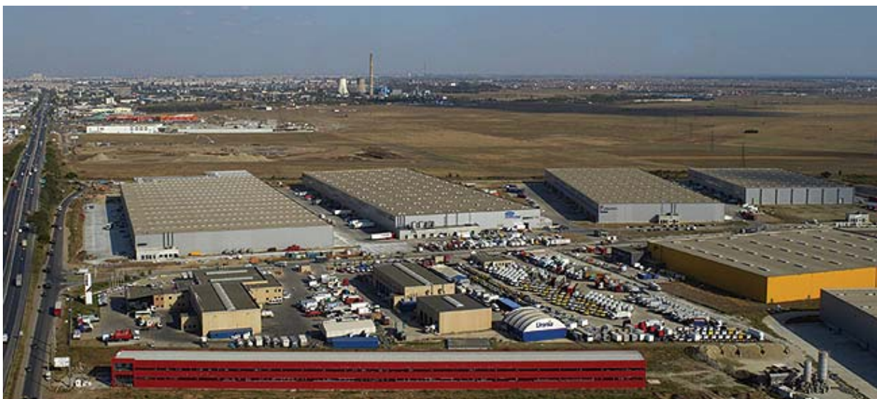
Logistics center in Romania: Europolis Park Bucharest
