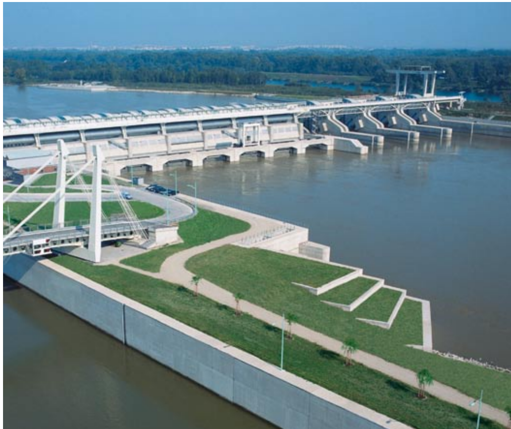
▲ Complete electromechanical equipment for large hydropower stations: Verbund-Austrian Hydro Power AG's Freudenu hydropower plant on the Danube, Austria.
