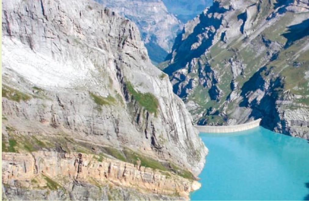
▲ Hydropower as renewable energy source: the Limmernboden reservoir in Switzerland, for which ANDRITZ HYDRO supplied, inter alia, the pump turbine ASB for the extreme head of up to 1,060 meters.
